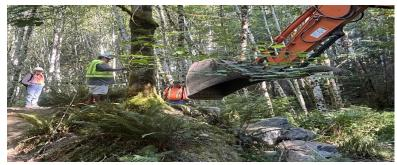
The old narrow gauge railroad grade was used to build a small weir with flow controls. Winter rains bring the level of the lake up enough to hold water for flows through the summer. In this way Coho fry can rear in healthy habitat for the first year of their life and then as smolts they swim out to the sea each spring.
